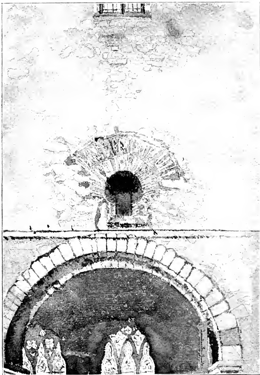
PART OF N. WALL OF NAVE.
